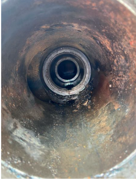
Figure 05-Scale in WT Kit after Well-5- RHS Choke Box
