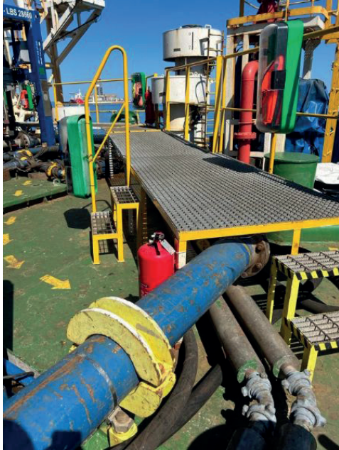
Figure 01-Walkways constructed in Well Test Area
