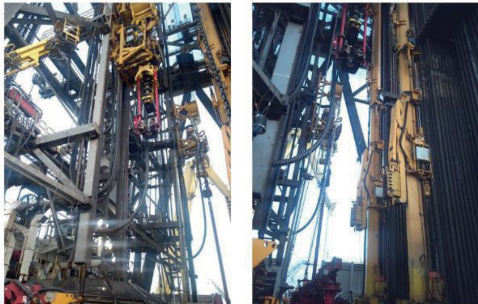
Figure 2 — Main & AUX TDS and Pipe Racking System
